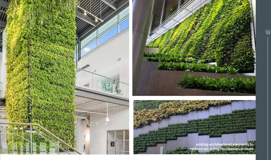
The benefits to these systems are the flexibility in large-scale design, engineered irrigation and fertigation controls that can be fine-tuned for the climate and season and the ability for the system to maintain the long-term growth of plant material for years to come.
