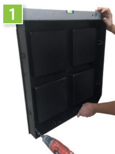
▪ Attach back frame to wall
